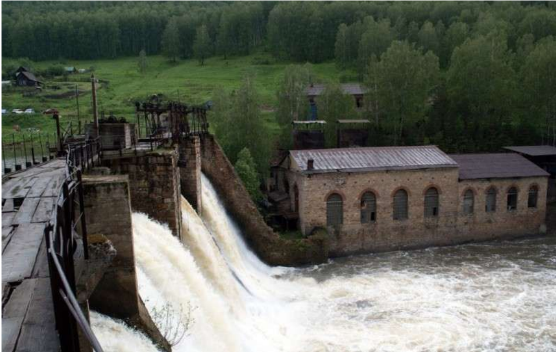
'Porogi' dam and workshops
