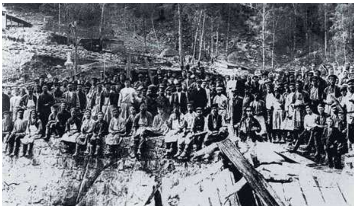
‘Porogi’ dam and plant construction, 1909
