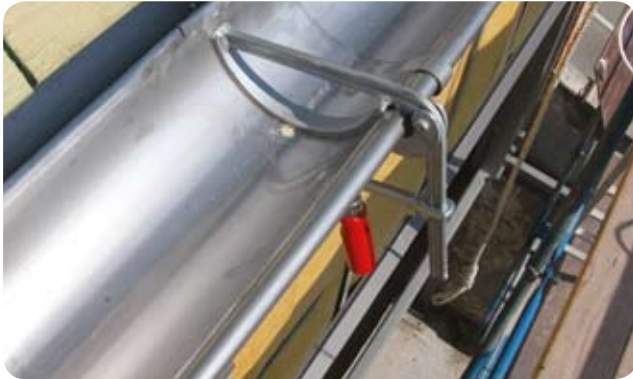
Bonding of guttering, tin-coated 430Ti.
