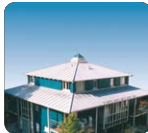
Grade 1.4510/430Ti (standing- seam technique), Ugine & Alz, Germany.
