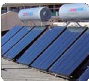
Grade 1.4509/441 (cylinder), Sun Tank and SASSDA, S. Africa
