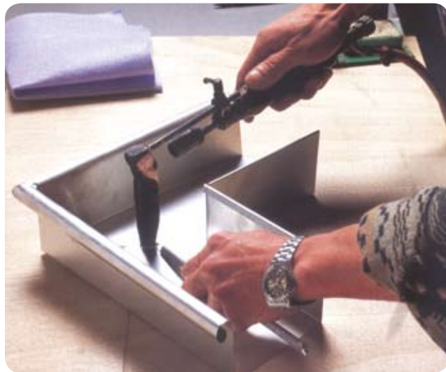
Soldering a gutter, tin-coated grade 430Ti.
